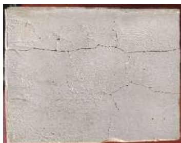
Fig.-5: Crack Formation in Compressive Strength Testing MOC Blocks of M0 Cementing Composition
